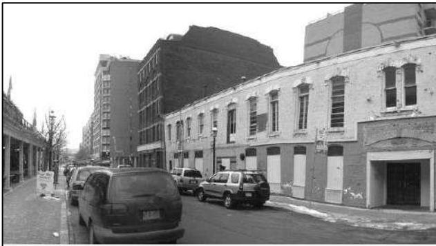
Neglected buildings on Market Street, 2011
